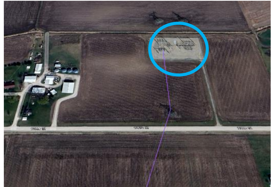
MidAmerican Energy's Sub 92 Substation near West Liberty in Muscatine County.
