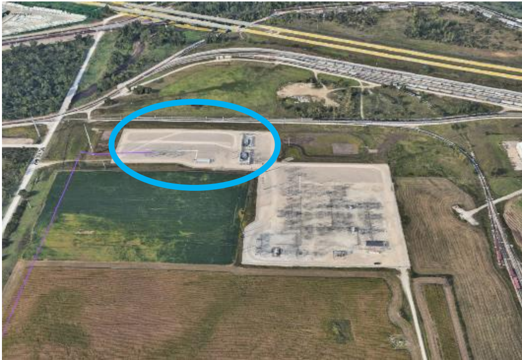
ITC Midwest's Beverly Substation in Cedar Rapids, Linn County.
